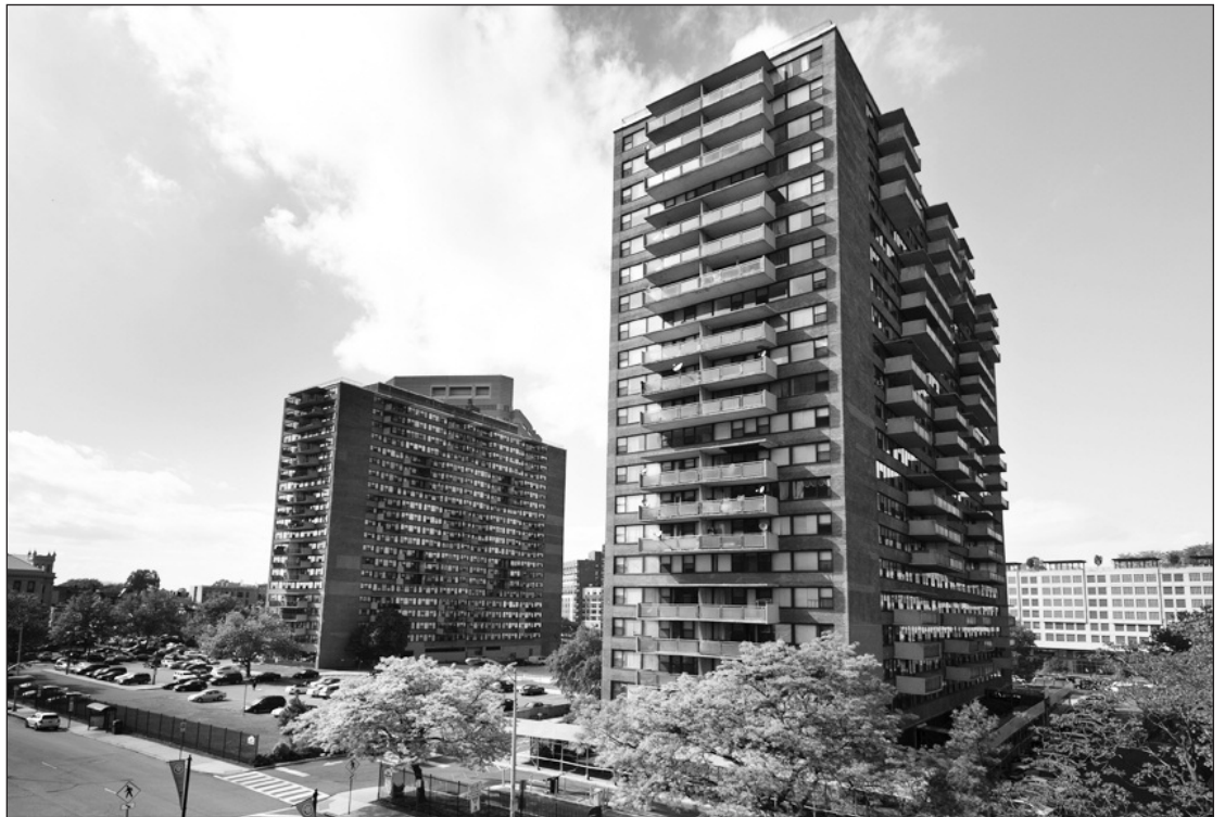
More than 26,000 cubic yards of chromium-impacted soil and debris located several feet below ground will be removed from the Metropolis Towers complex.
